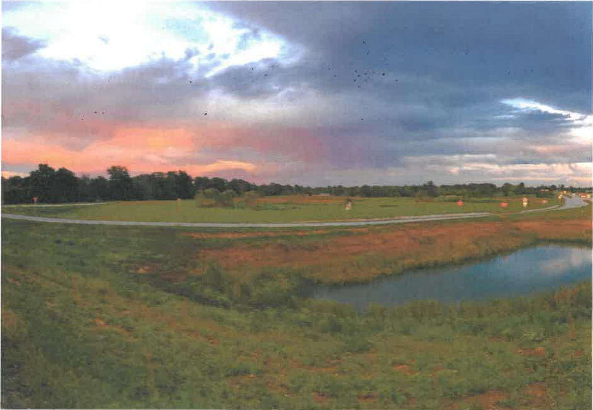
Image: Karst geology and sinkholes terminated development of a 42-acre parcel (above) on the northwest corner of the Highway 60 and Farm Road 253 interchange.
