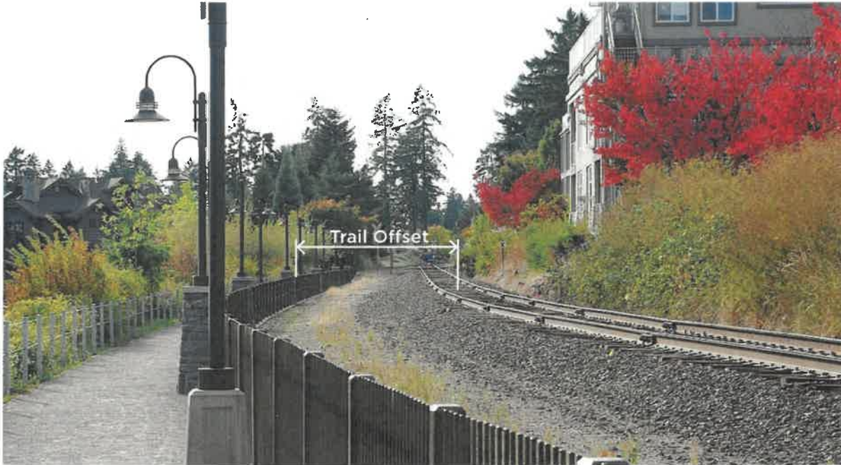
Image: Railroad companies typically require fencing and offsets from railways for parallel paths.
